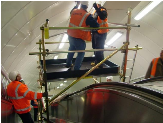
Above Escalator Maintenance
