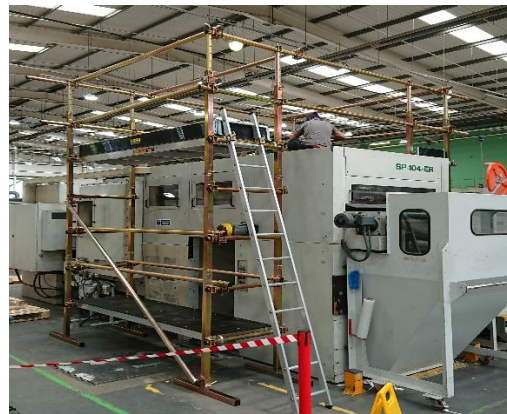
Building Around Machinery
