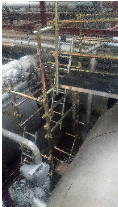
Toe boards added before use.
