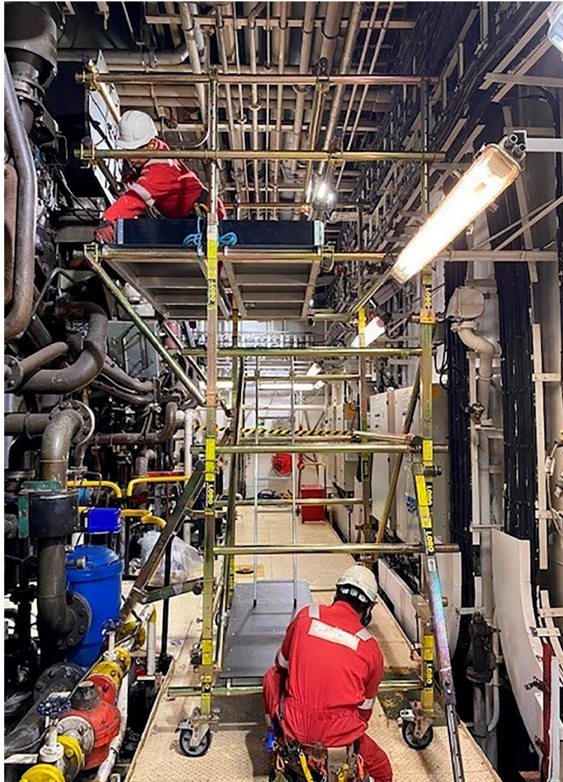
Figure 1 Engineers accessing engine turbocharger via LOBO System.
